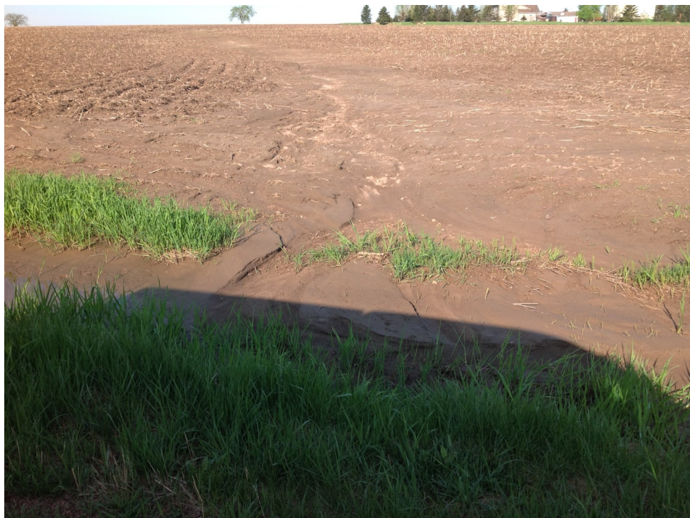
Two feet of sediment in Road Ditch
