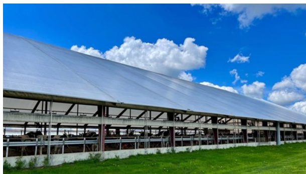
Figure 2. Split sidewall curtains help regulate airflow rates without causing a draft for the cows. (Photo: Nesli Akdeniz)
