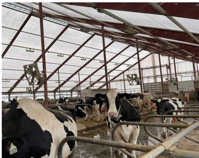
Figure 4. Naturally ventilated fabric dairy buildings. Note the steep 6:12 roof pitch. (Photo: Nesli Akdeniz)
